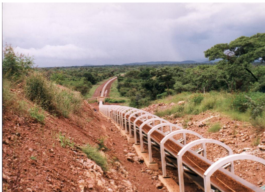
Figure 1 - Looking Toward Direction of Flow at 2300m chainage
