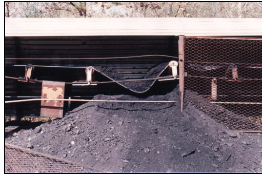
Figure 15 - Sag Spillage Stockpile
