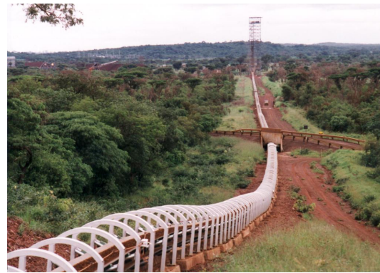
Figure 2 - Looking at Take-up Tower (Opposite Figure 1 Vantage)
